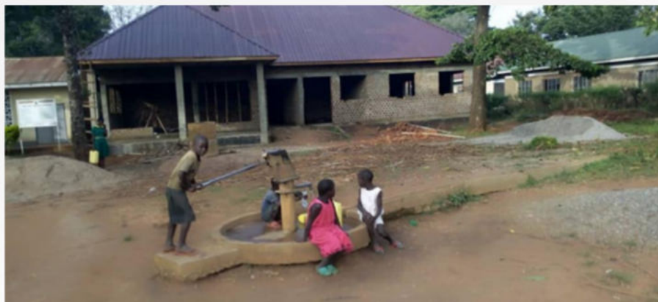
The New uncompleted Maternal and Child Health unit constructed by the Community of Lumino.
